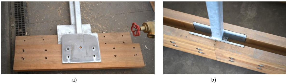
Fig. 4 – Splice connection: a) steel post with link steel and timber elements; b) beam ready for erection.
